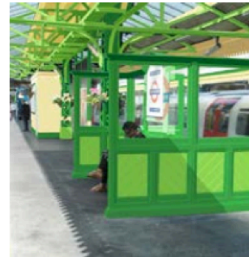
Turnham Green painted timber platform screens.
