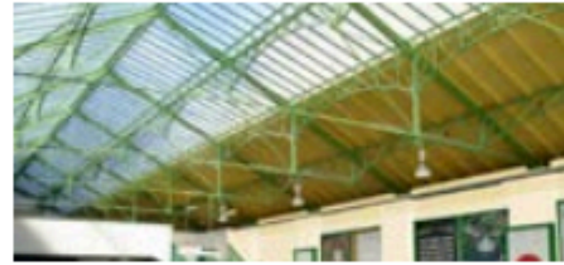
Roof trusses and framework (Ealing Broadway)
