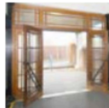
Decorative timber work Door (Brent Cross)
