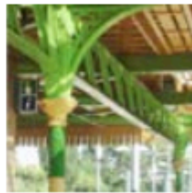
Cast iron Canopy supports (plat)
