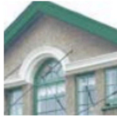
Timber Painted cills/window frames/ external architrave
