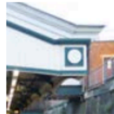
Platform canopy detail (Colindale)
