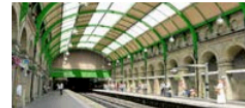
Notting Hill Gate Cast iron painted arch and glazed roof
