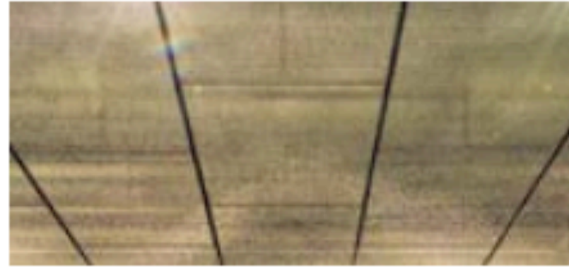
Stainless steel woven mesh ceiling
